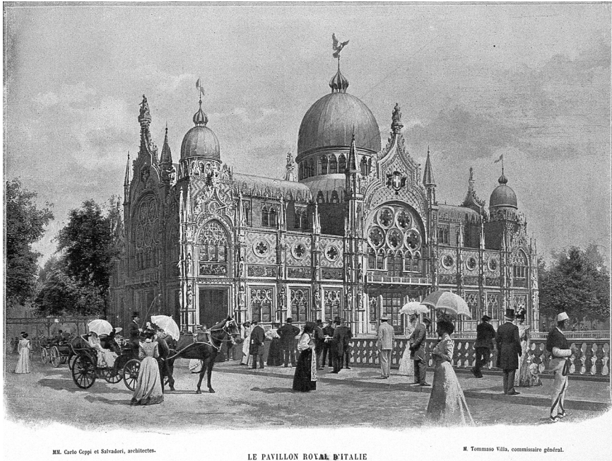
Figure 1.3 View of the Italian Pavilion from the Pont des Invalides at the 1900 Paris World Exhibition. Source: Baschet (1900b), provided by Universitätsbibliothek Heidelberg, https://digi.ub.uni-heidelberg.de/diglit/baschet1900/0110 .
